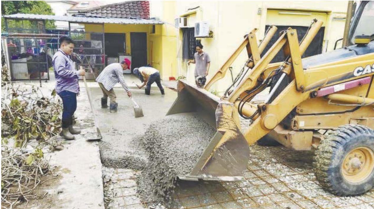
Volunteers working on the improvements at the home.
